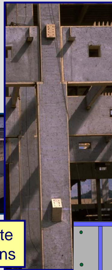
concrete encased sections
