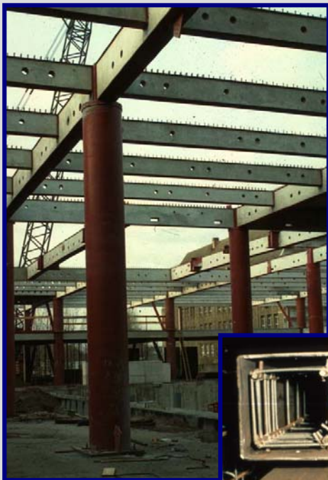
concrete filled hollow sections
